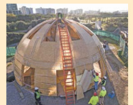
2024: Construction of first outer layer.
