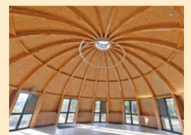
June 2024: The completed Dome roof.
