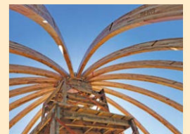
2023: Skeleton of curved beams constructed to form roof.
